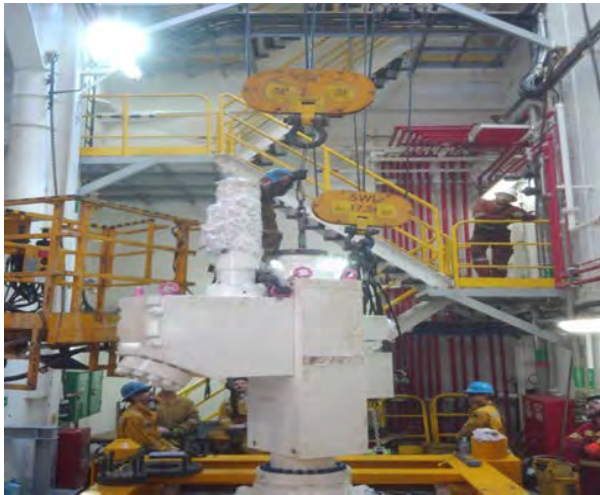
FIGURA 28: OBSERVA PROSESU HATUN W12-MASS TREE FIGURA 29: OBSERVA WELL TEST POSO W12
